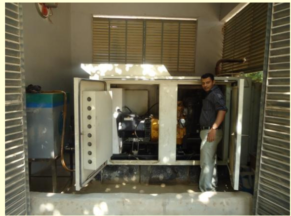
Mr. Ubaid working on MCN generator
