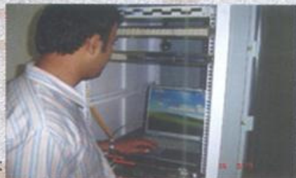
Project Engineer Configuring the network wireless bridges at the Data Center
